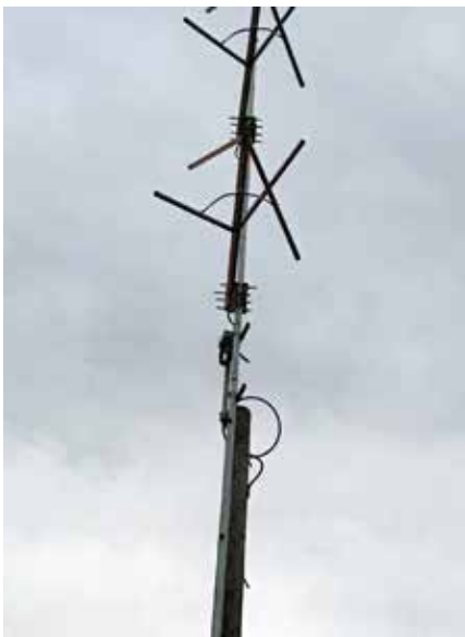
Completed antenna installation.
