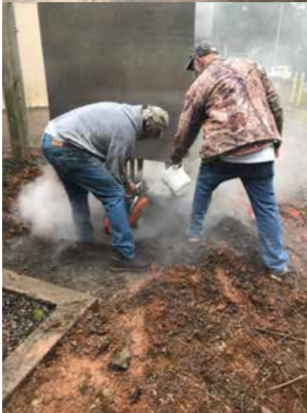
Steve and Albert cutting asphalt.
