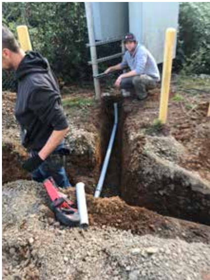
Electricians installing conduit.
