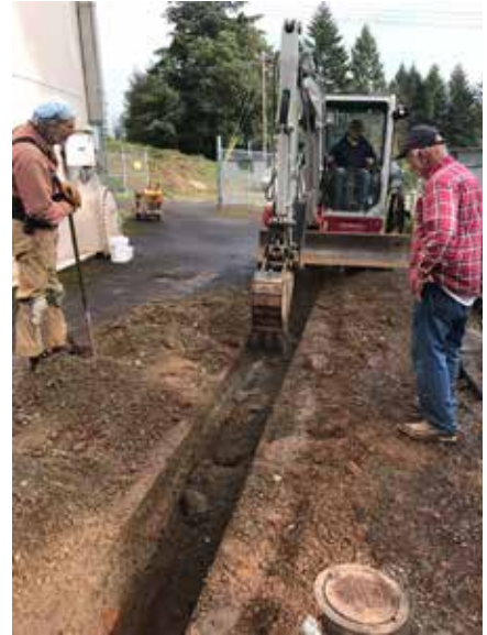
Mouseman and Albert checking the ditch.
