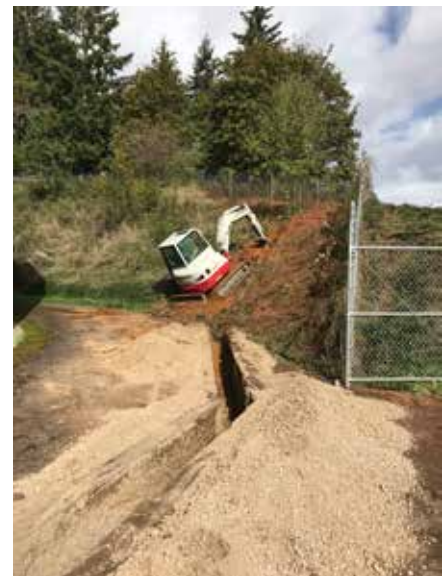
Steve precariously digging the trench
