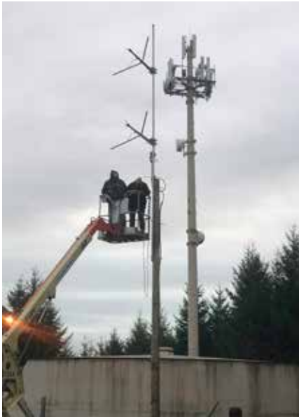
Mouseman and Jay securing coax tower.
