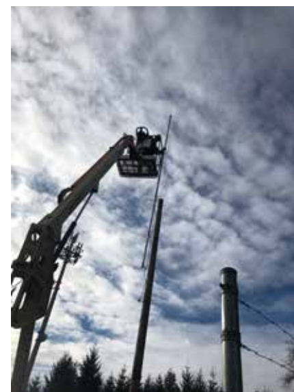
Jay attaching antenna pole to tower.
