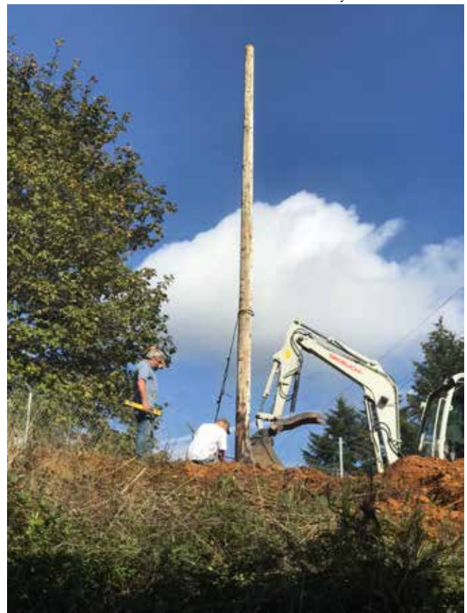
Steve and Albert setting the monopole.
