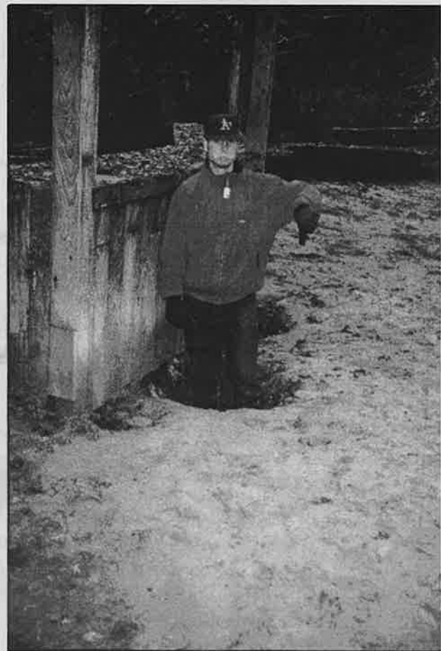
Caretaker Andyman points out negative effects of solid booth fronts and river erosion at the Bangkok Grill booth on River Loop.
